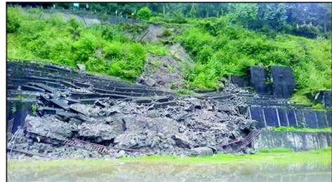
The galleries at the Public Ground, Mangon, in North Sikkim have collapsed under the impact of a landslide. The public gallery walls were already cracked at several places at the time of construction and expansion work of the ground. Now it's the season of rainfall and natural calamities and the gallery walls have not withstood the pressure. --- DEEPAK SHARMA
